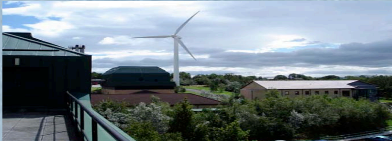
Figure 11: Antrim Area Hospital's V47 660 kW Vestas wind turbine. As suggested by its model number, V47, this particular Vestas turbine has a rotor diameter of 47m. Source: Sustainable Development Commission n.d.
