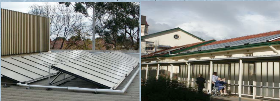
Figure 14, 15: Solar assisted hot water systems for the Repatriation General Hospital in Adelaide. Through these solar collectors (left) and other initiatives such as natural gas burners, 56% of the hospital's heating requirements are now powered with alternative energy.
