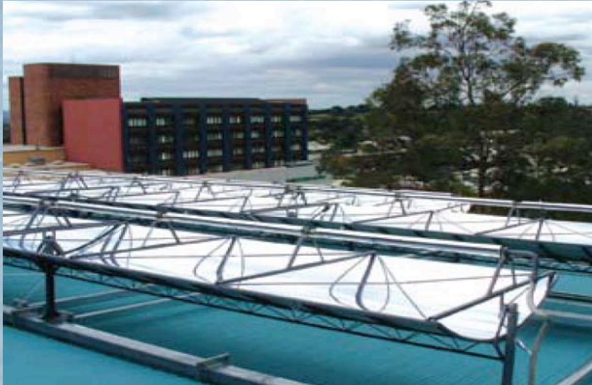
Figure 16: The Ipswich Hospital thermal solar collector field is powered by 43 solar collectors on top of its parking facility. Weather dependent, the field generates approximately 255kW/h.
