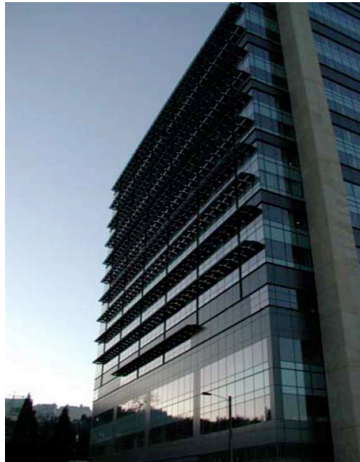
Figure 13: Photo of the south façade of the Centre for Health and Healing at OSH, with its sunshades that incorporate solar PV panels.
