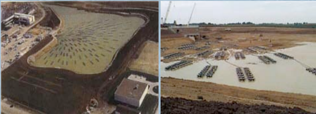
Figure 9, 10: Artificially constructed lake in West Burlington that acts as the 'heat exchange field' for the Great River Medical Centre's geothermal heating/cooling system. While still in construction phase, the devices shown on the lake floor are the grids and pipe coils, or heat exchangers, which will ultimately transfer heat from the water at the bottom of the lake to supplement the centre's heating/cooling requirements. Sources: 9, Alliant Energy n.d 10, Sherman Health n.d.
