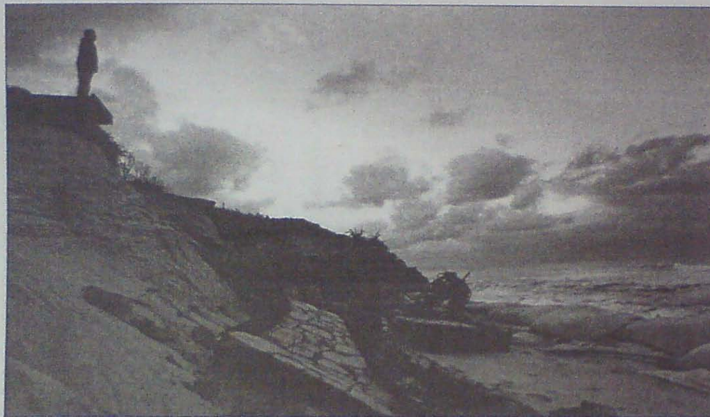
Byron Bay . . . the beachfront has suffered massive erosion after recent storms.
